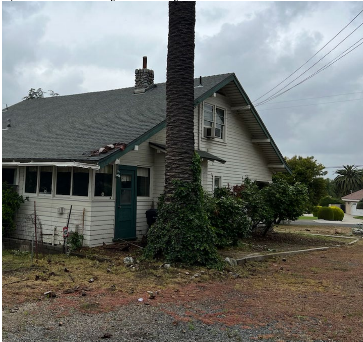
Figure 6. North facade, looking southwest
