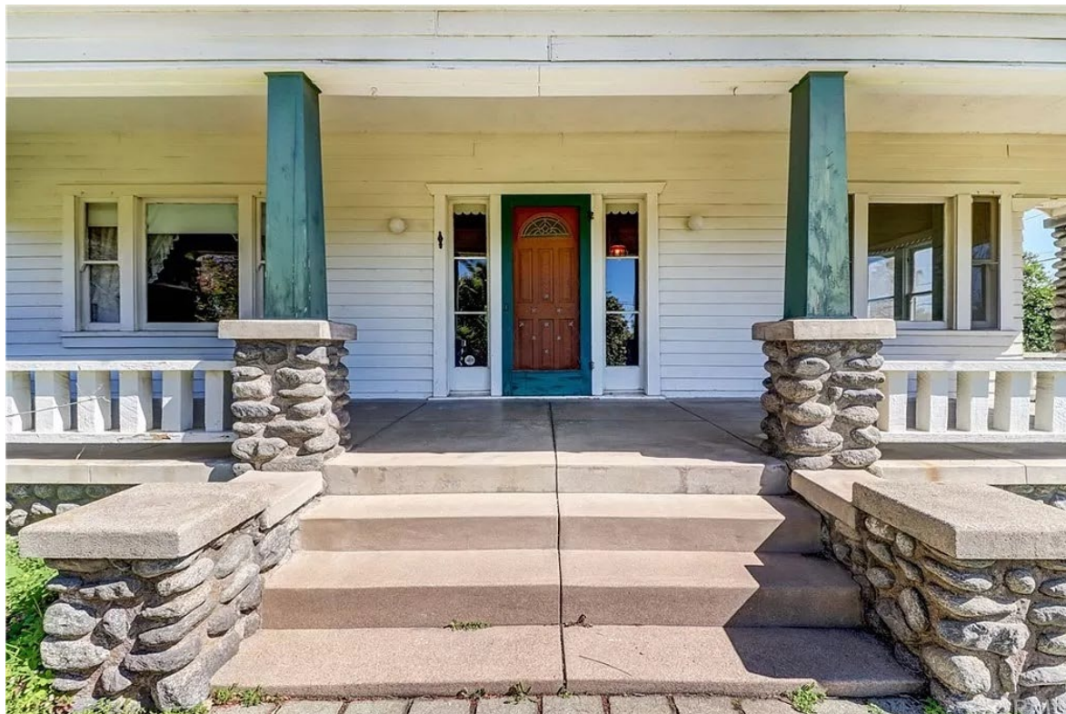
Figure 5. West facade and porch with stone and wood tapered piers, view east
