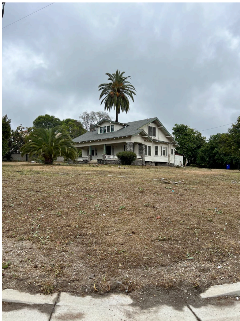
Figure 1. Main house as it appears from the street looking NE
